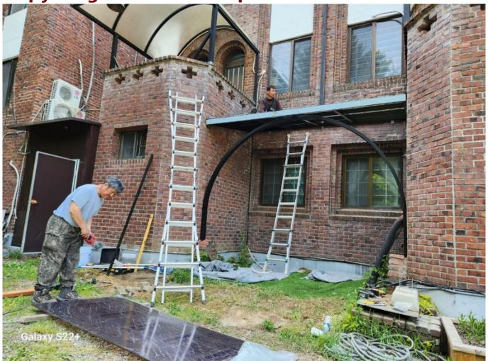
From May 14th to 22nd, the monastery's exterior walls were repaired by filling in gaps, waterproofing, and installing eaves to prevent water flow. The necessary repairing work has resolved a long-standing problem of water leaking through the interior walls and into the basement.
