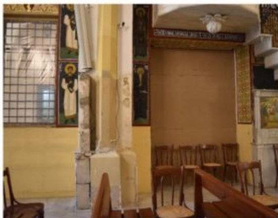
Openings rehabilitation - before
