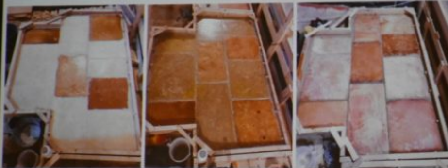
Flooring samples in situ
